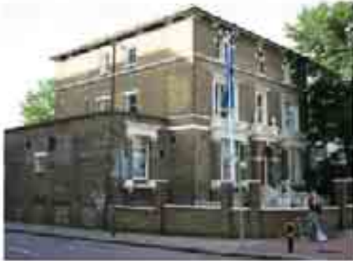
Delta House 8kW Packaged System
